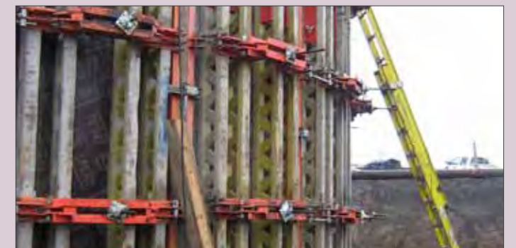
TaigaNova Eco-Industrial Park under construction
